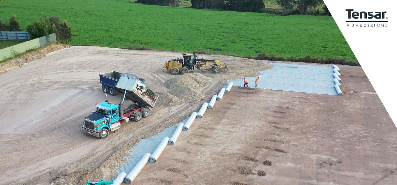
Laying and compacting the first layer of mechanically stabilised layer on the subgrade
